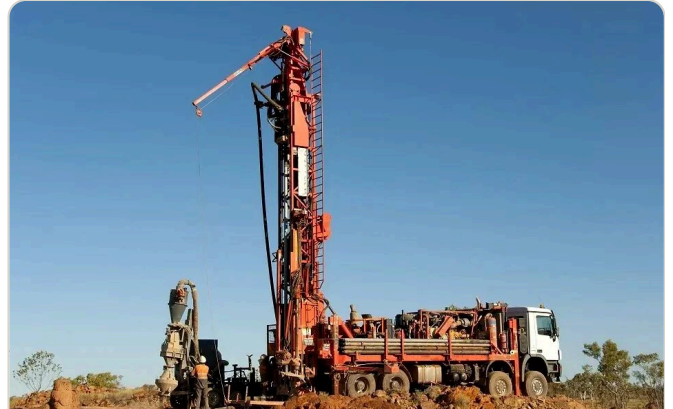
Reverse-circulation rig, truck-mounted, operated by our own crew.
